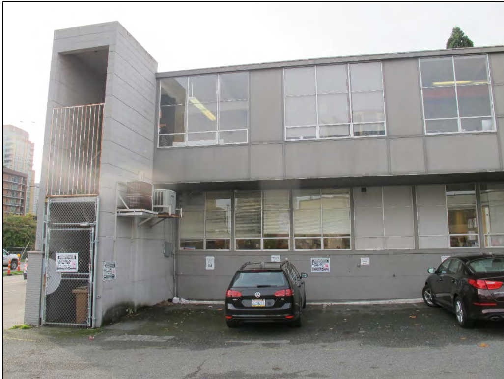
Fig. 21 – (2016) North elevation, east part
