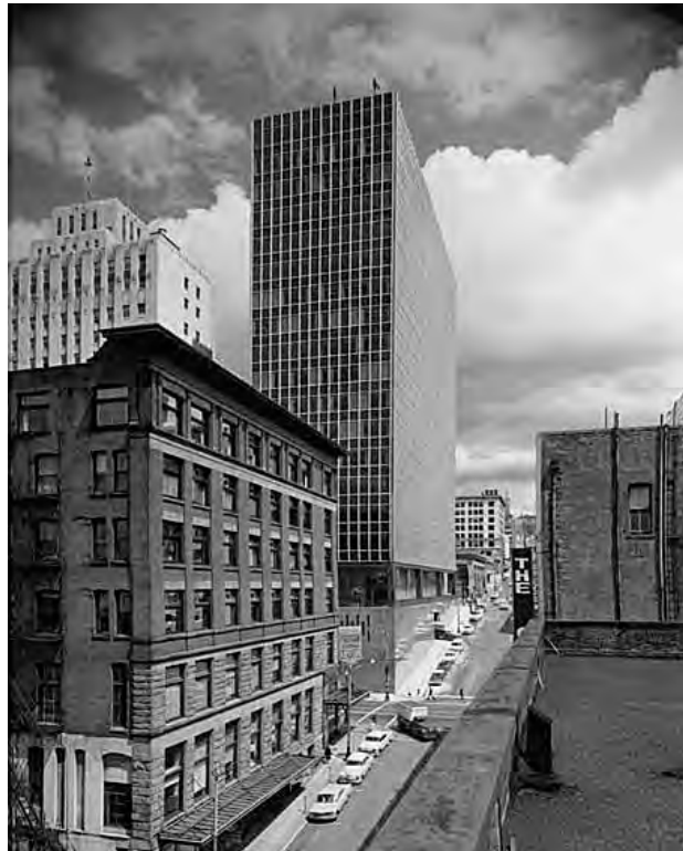
Fig. 80 – Curtain Wall: Norton Building (1959, Bindon & Wright, with Skidmore Owings & Merrill). The Norton Building is a designated Seattle landmark. (MOHAI DMA0075)
