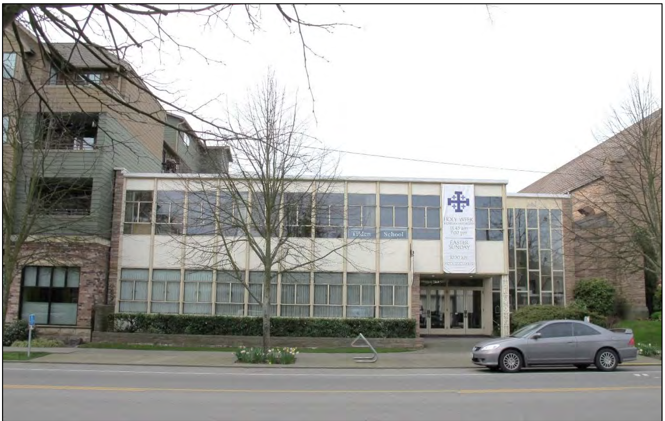
Fig. 78 – Curtain Wall: First Lutheran Church school, (Durham Anderson & Freed, 1957) at 4105 California Avenue Southwest
