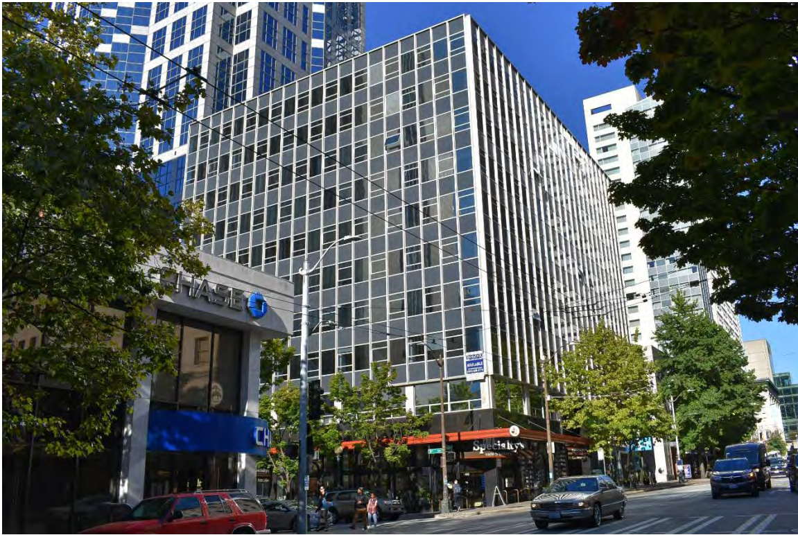
Fig. 79 – Curtain Wall: Logan Building (1959, Mandeville & Berge)
