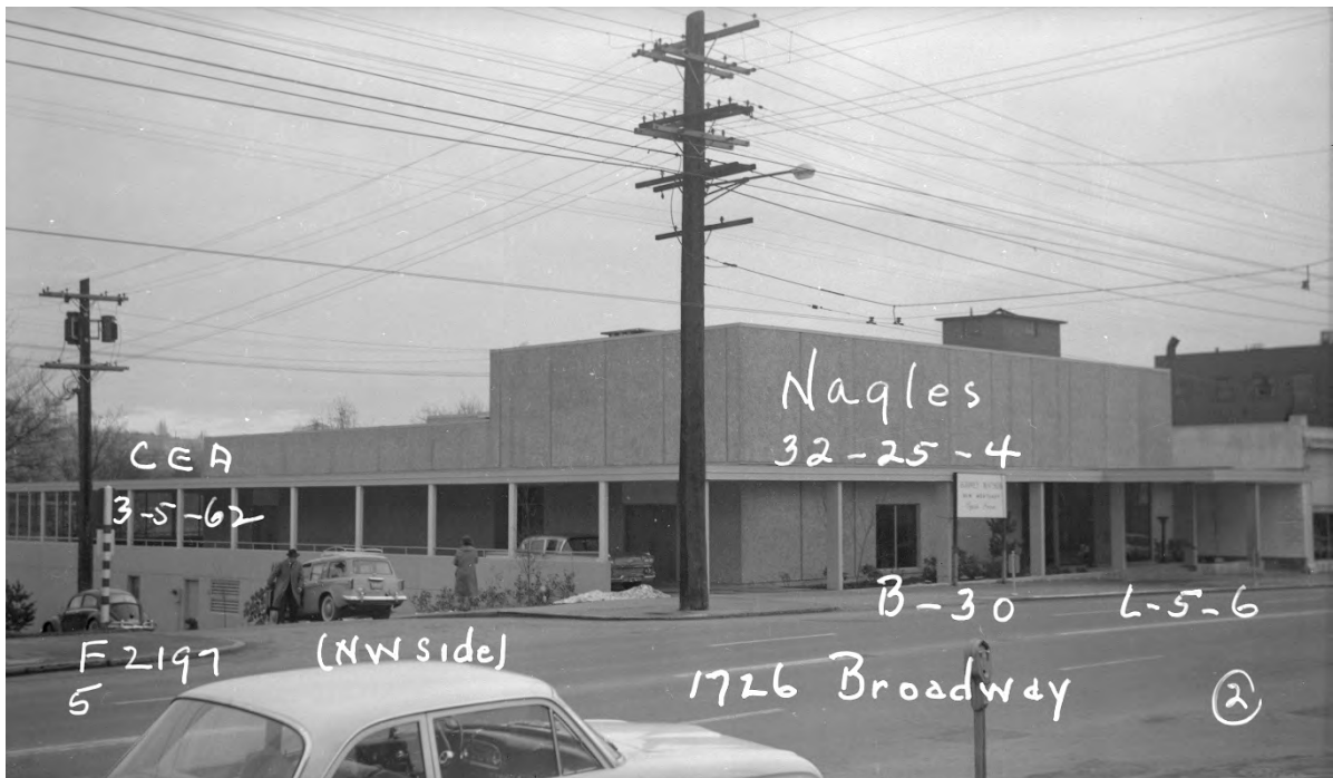
Fig. 74 – E. F. Shuck Construction Company: Bonney-Watson Funeral Home (Bain & Overturf, 1962). Constructed by the E. F. Shuck Company, as was the subject building. (PSRA)
