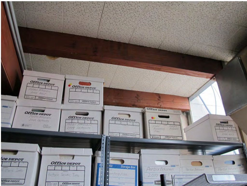
Fig. 38 – (2016) Interior, second floor storage room, showing original finishes.
