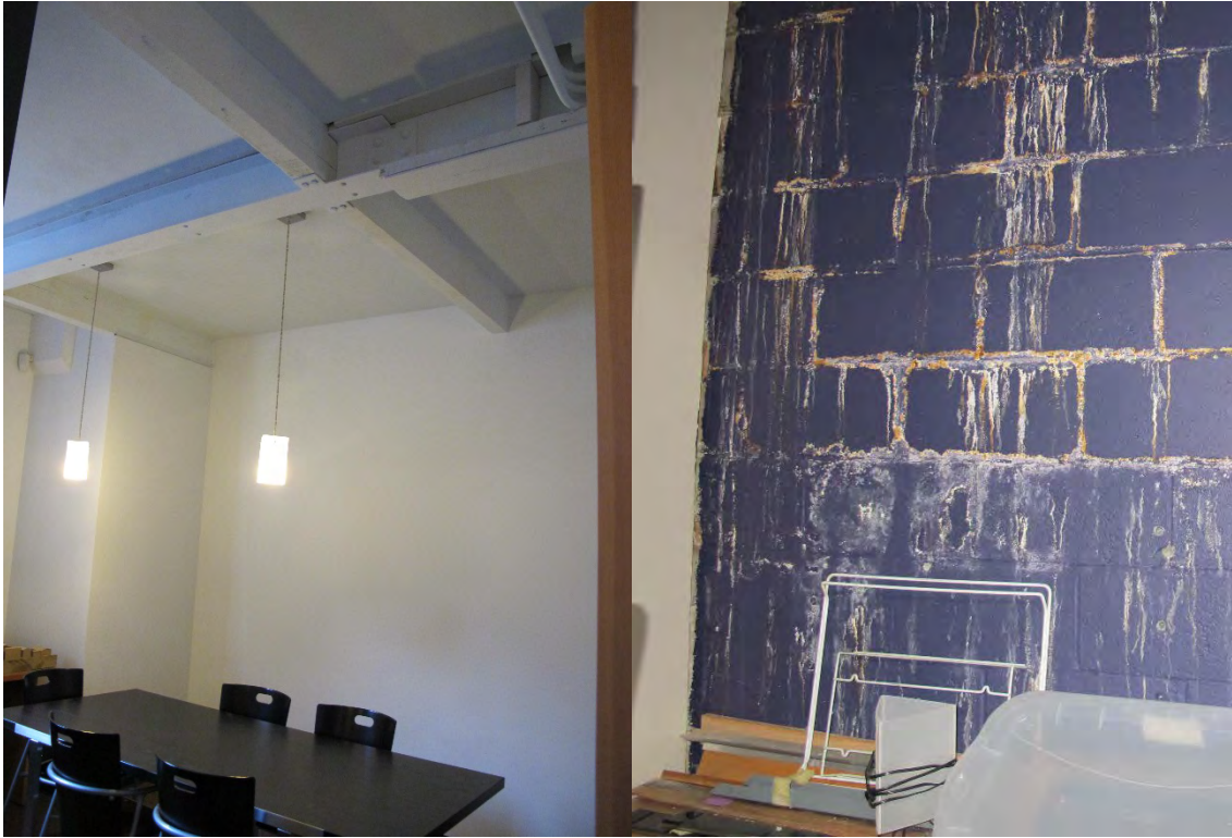
Fig. 39 – (2016) Interior, second floor, showing roof structure and concrete block wall
