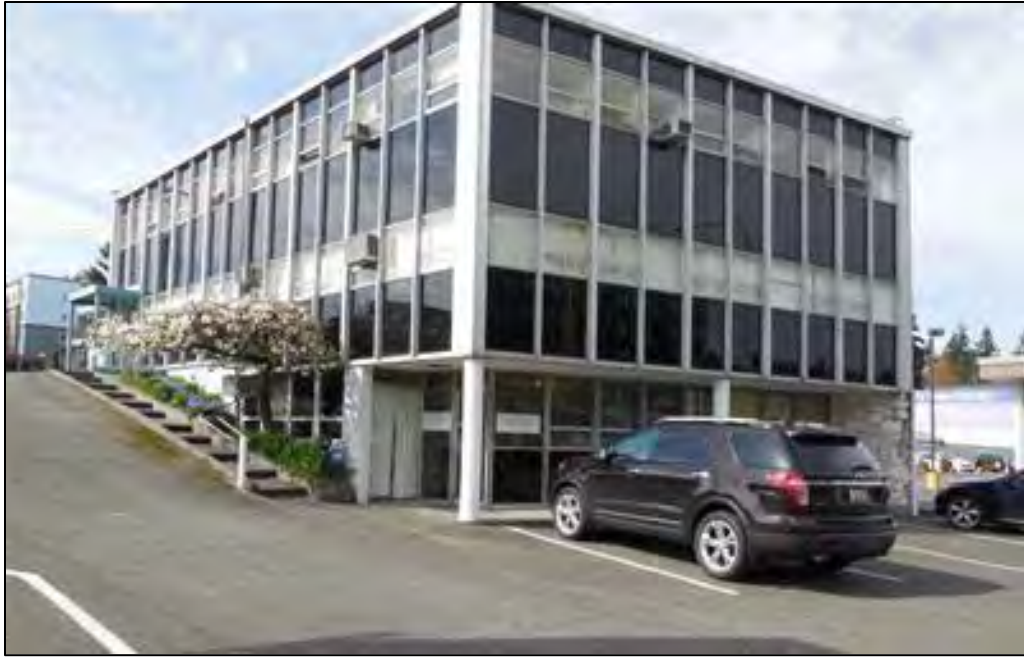
Fig. 81 – Curtain Wall: Office building at 12733 Lake City Way (1960) (King County Tax Assessor)
