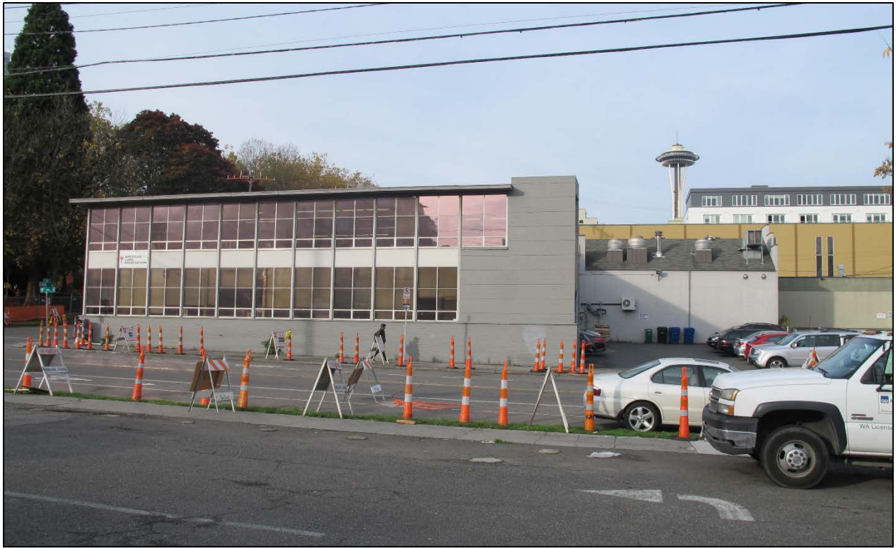
Fig. 17 – (2016) East elevation, facing 9 th Avenue North
