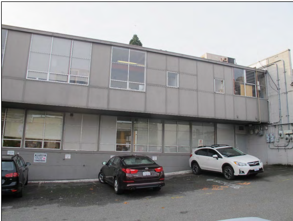
Fig. 22 – (2016) North elevation, west part
