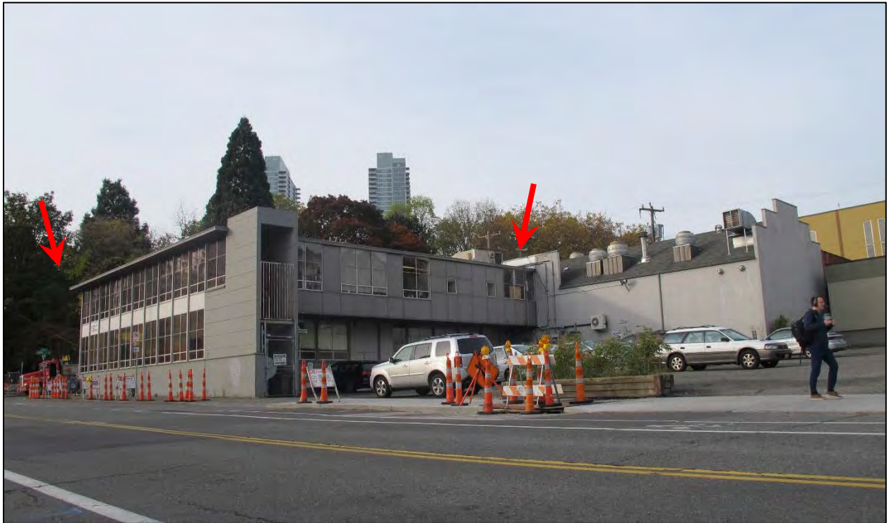
Fig. 18 – (2016) View of building from the northeast; subject building is between two arrows.
