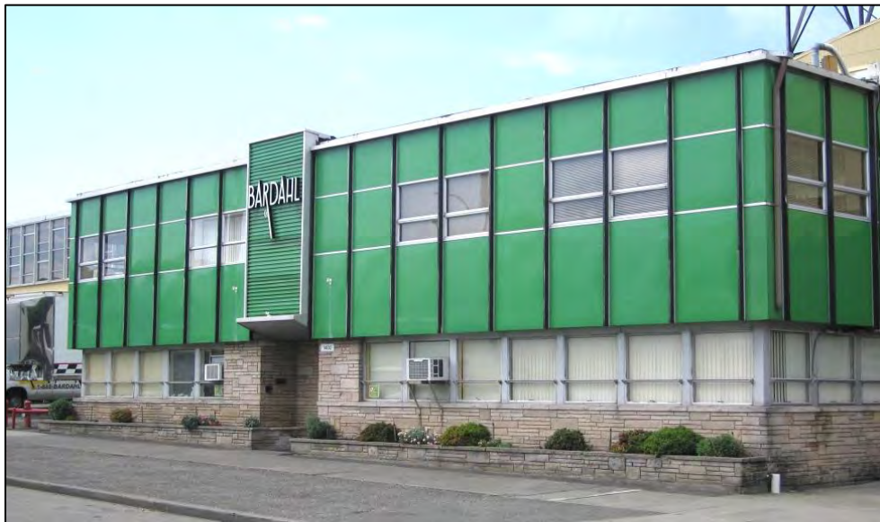
Fig. 76 – Curtain Wall: Bardahl Manufacturing Company, Ballard (1952) (DAHP)
