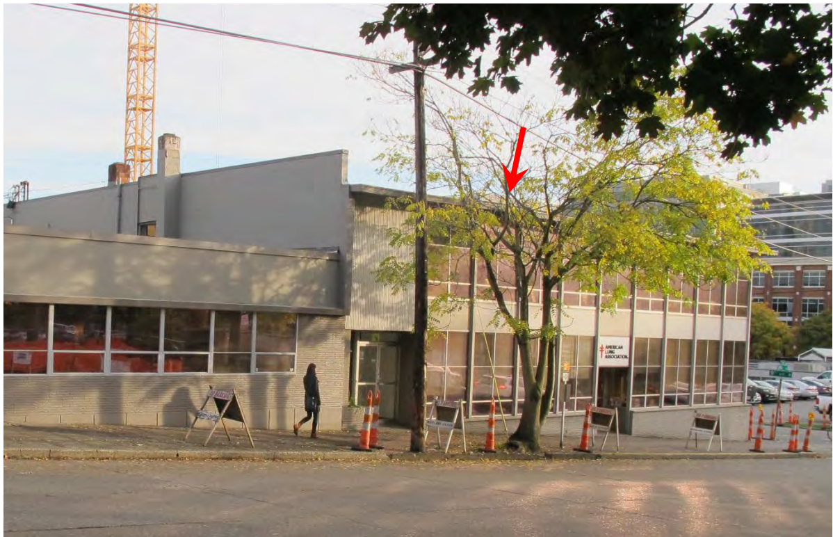
Fig. 14 – (2016) Context: View from Denny Park, subject building indicated by arrow.
