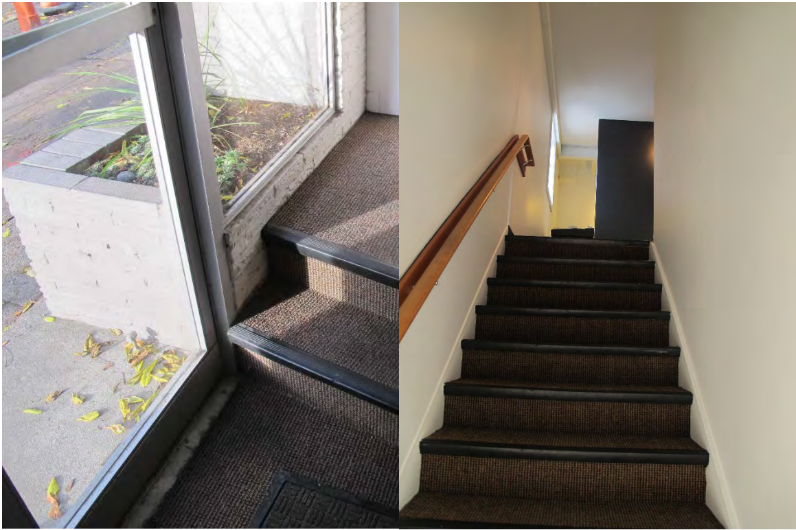
Fig. 31 – (2016) Stair vestibule to second floor
