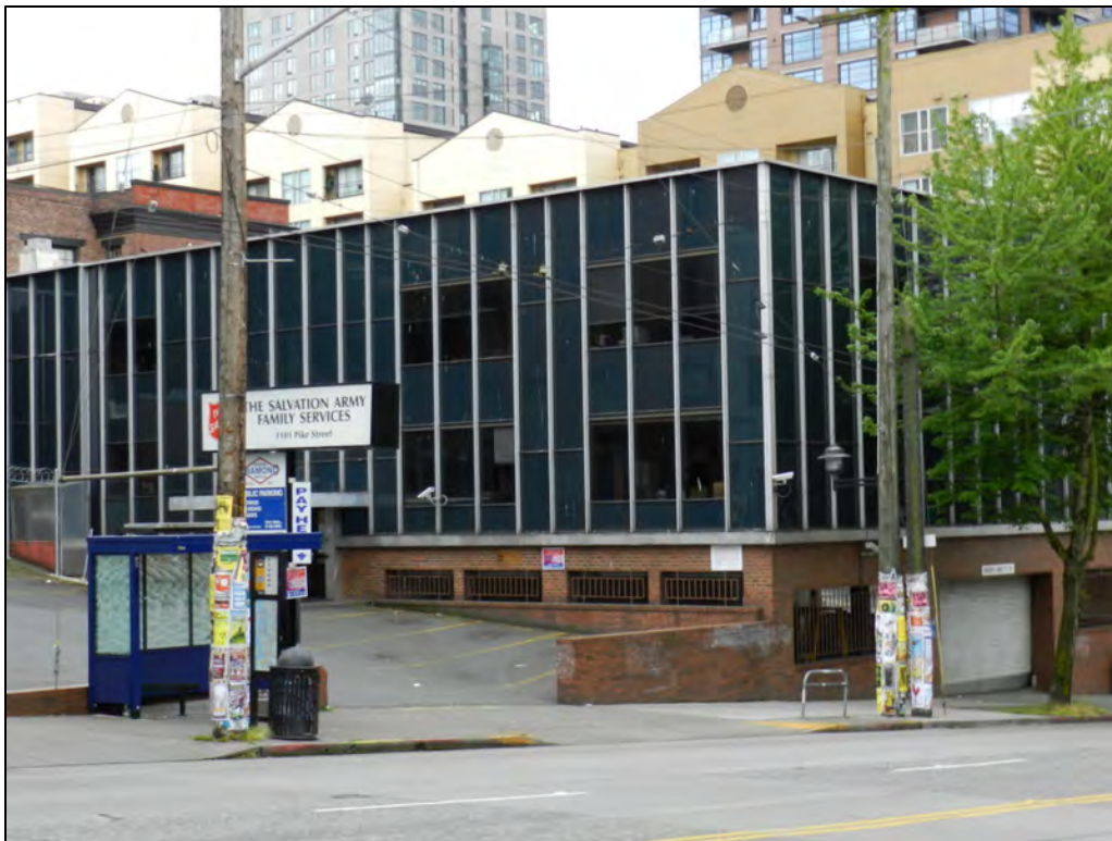
Fig. 84 – Curtain Wall: Salvation Army at 1101 East Pike (1964) (DON)
