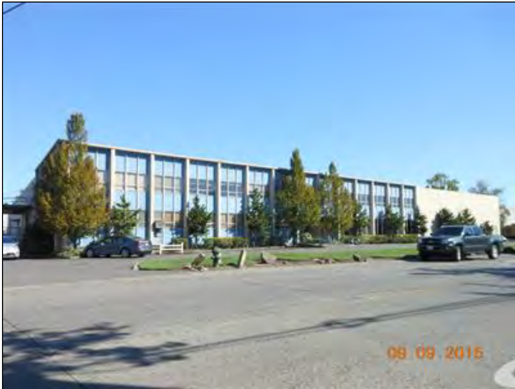
Fig. 83 – Curtain Wall: Washington State Ferries building at 6000 6 th Avenue South (1963) (King County Tax Assessor)
