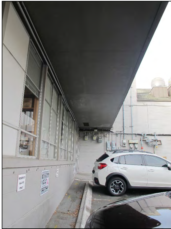
Fig. 23 – (2016) North elevation, looking west
