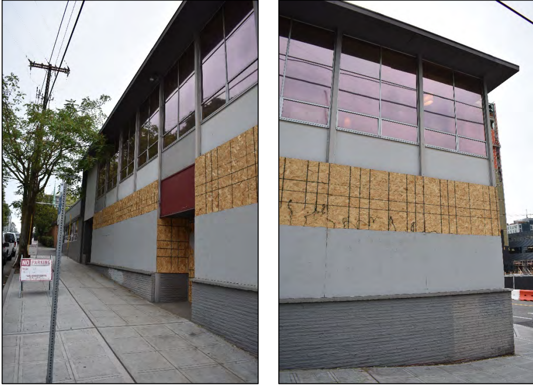
Fig. 9 – Detail, south elevation
